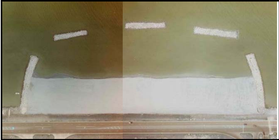
Figure 3. Post-construction aerial view of initial salient development taken on 08/26/2001 (Lanmon Aerial Photography, Inc.).
