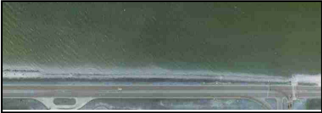
Figure 1. Post-demolition/preconstruction aerial view taken on 05/02/2001 (Lanmon Aerial Photography, Inc.).
