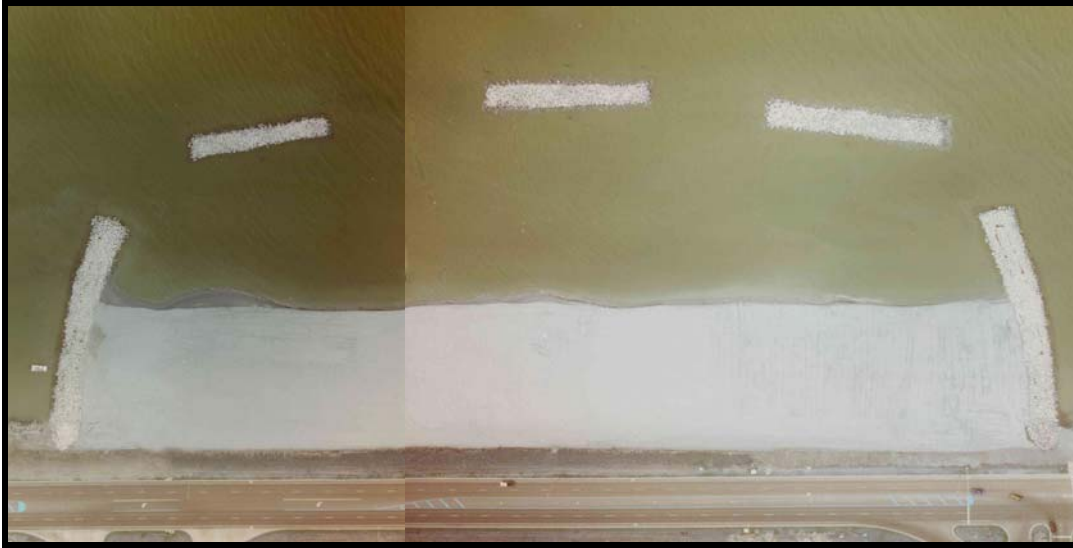
Figure 10. Salient development in the lee of DBWs occurred immediately after construction 08/26/2001.
