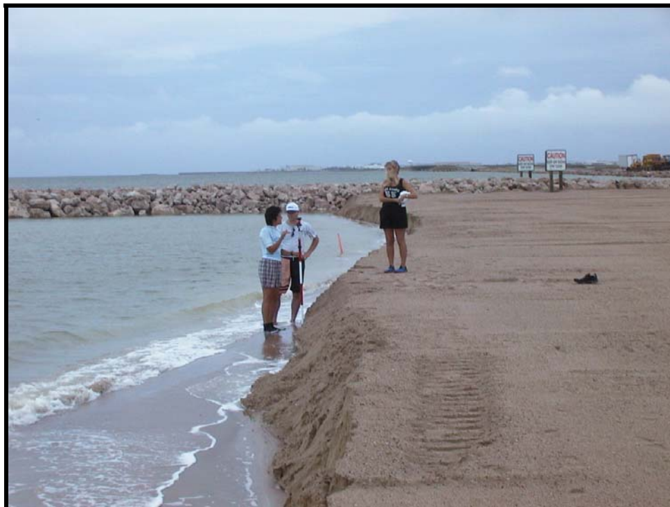
Figure 7. Nearly vertical wall of sand along shore immediately after beach placement 08/31/2001.
