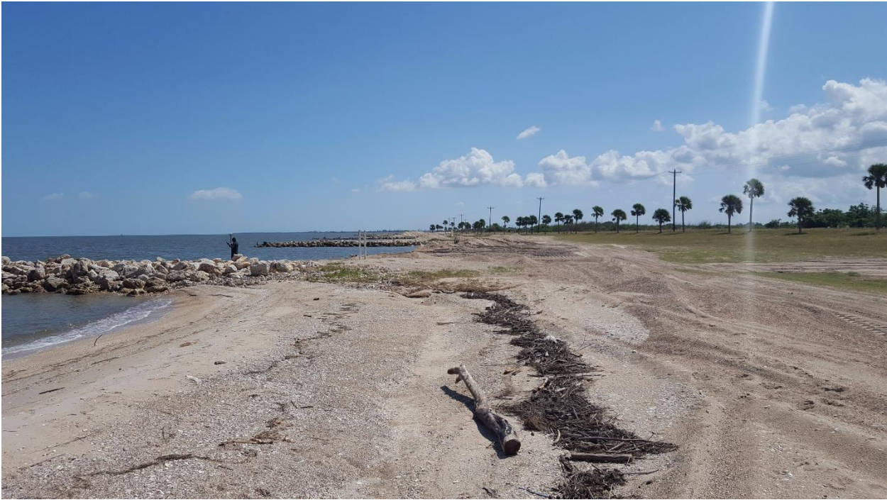
Southeast of STA 47+00
