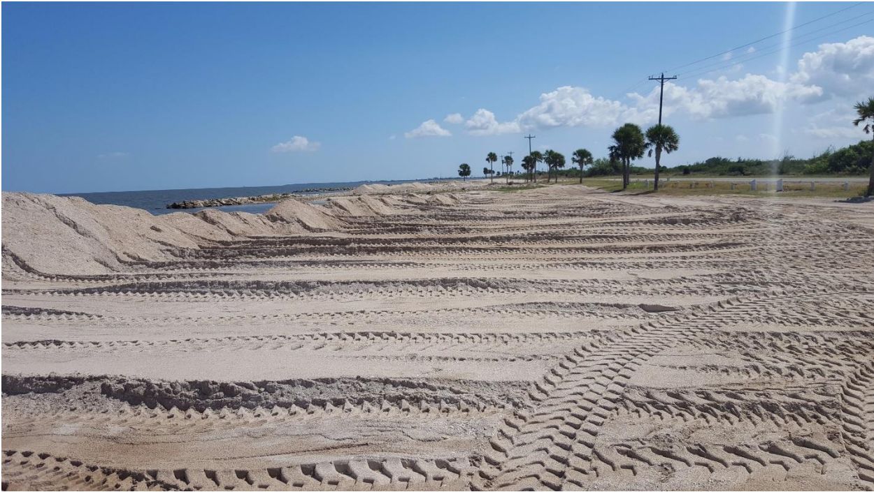
Southeast of STA 40+00
