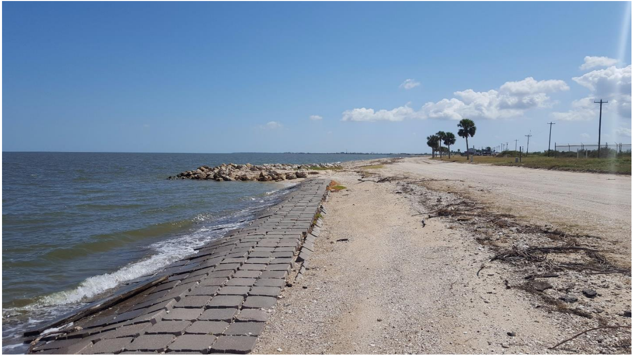
Southeast of STA 27+00
