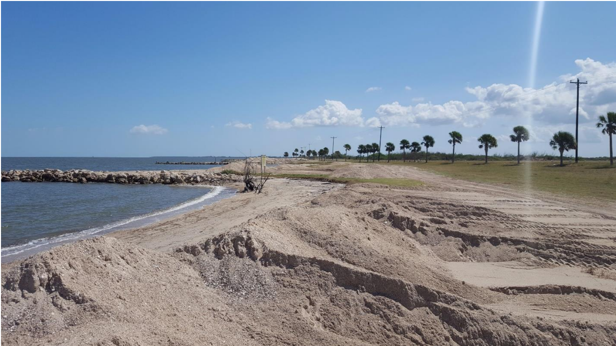
Southeast of STA 45+00
