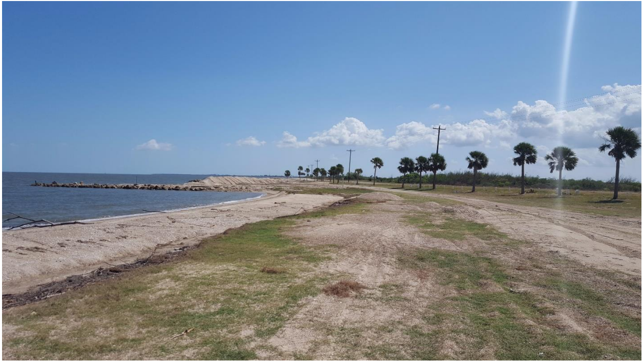
Southeast of STA 43+00
