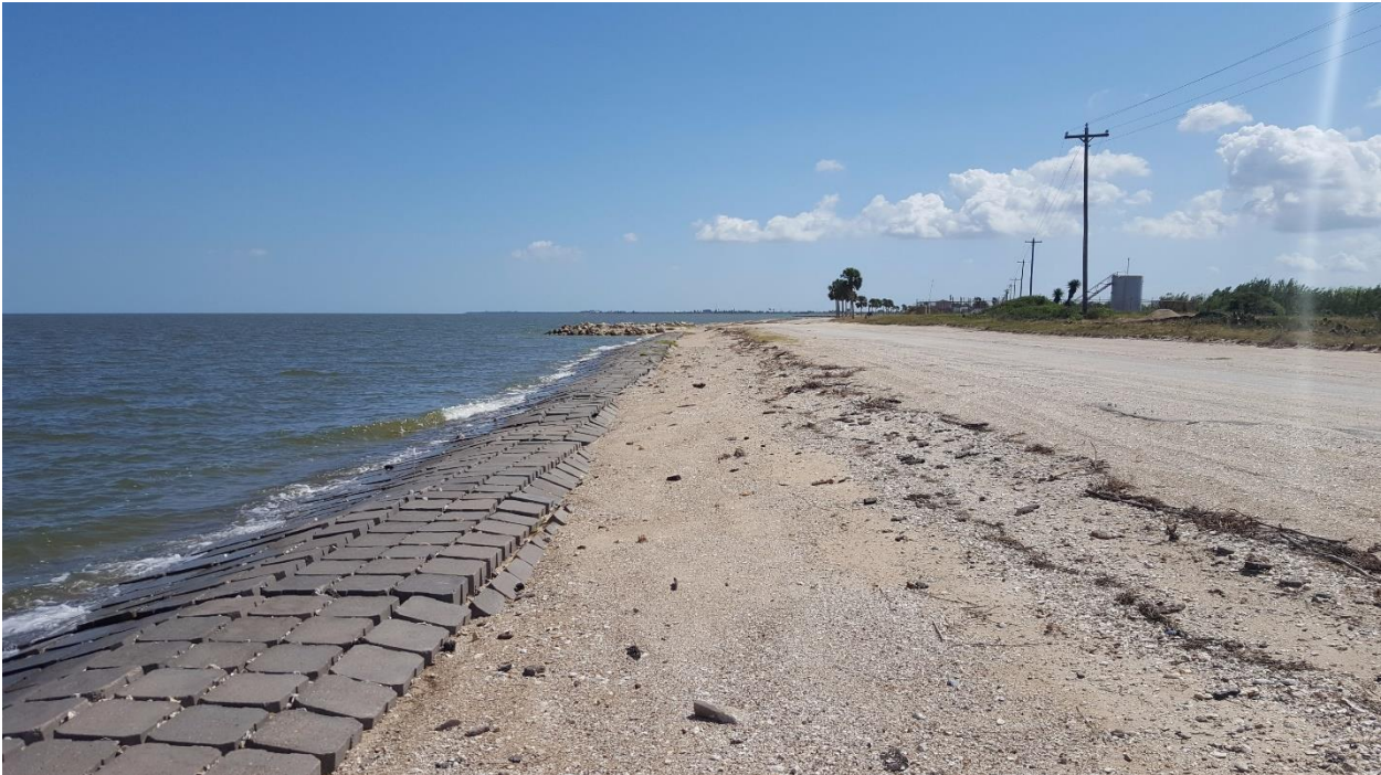
Southeast of STA 29+00
