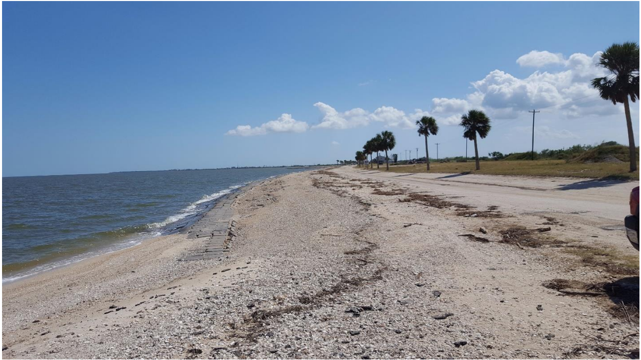
Southeast of STA 25+00
