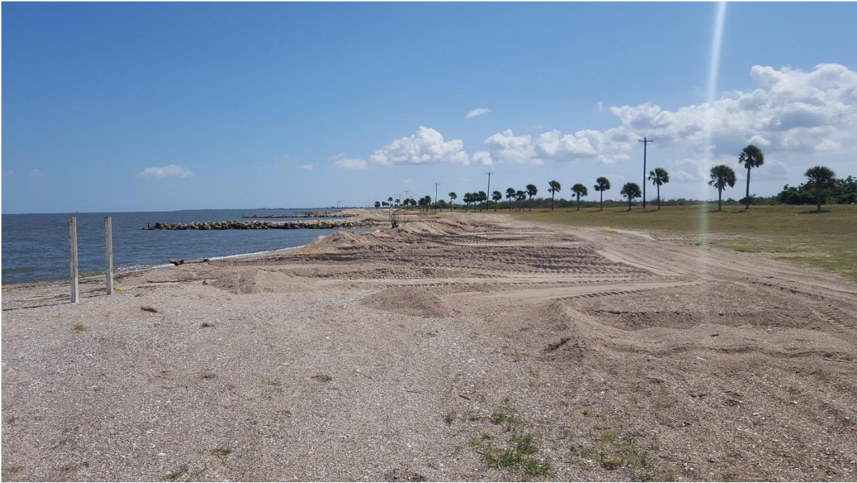
Southeast of STA 46+30
