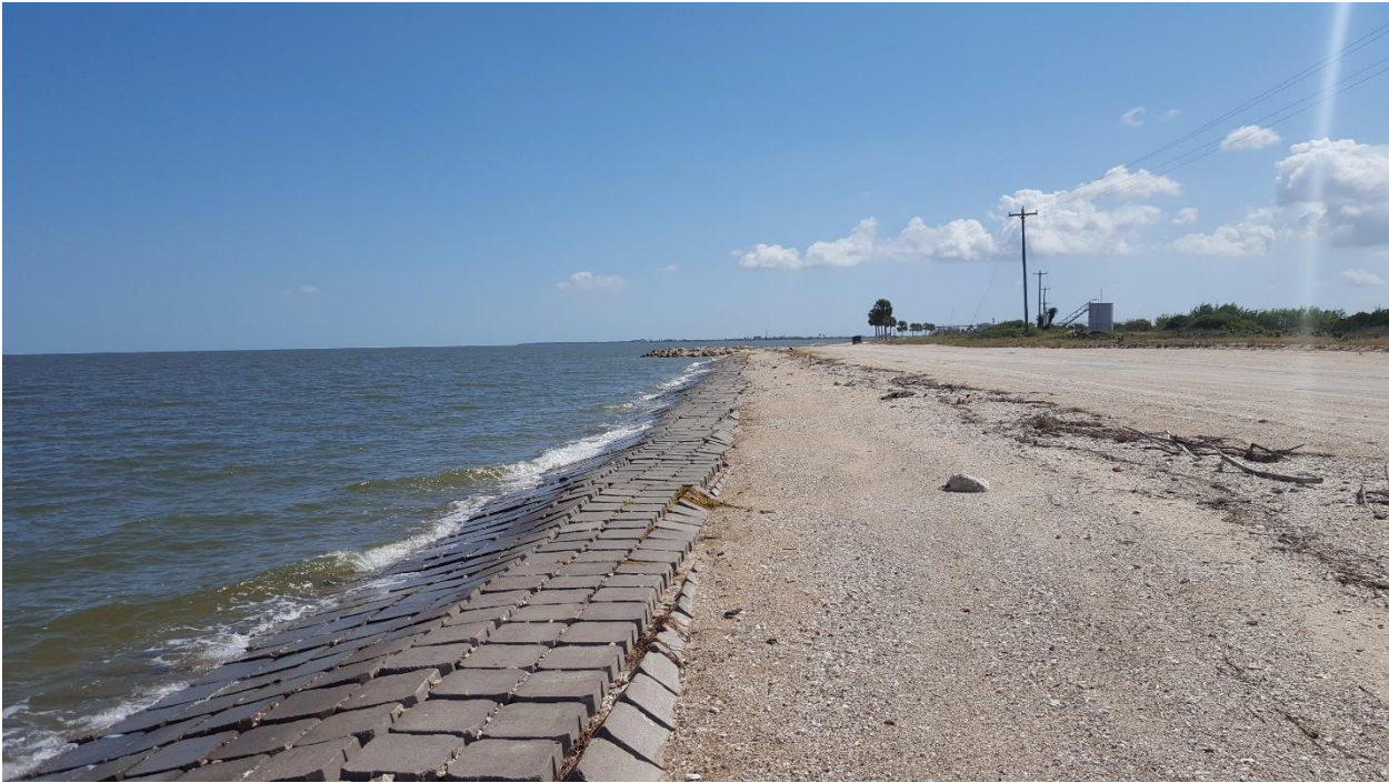
Southeast of STA 31+00
