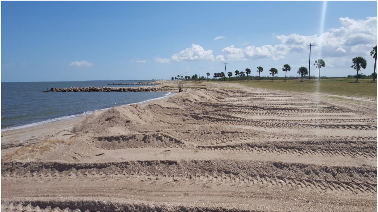
Southeast of STA 45 +80
