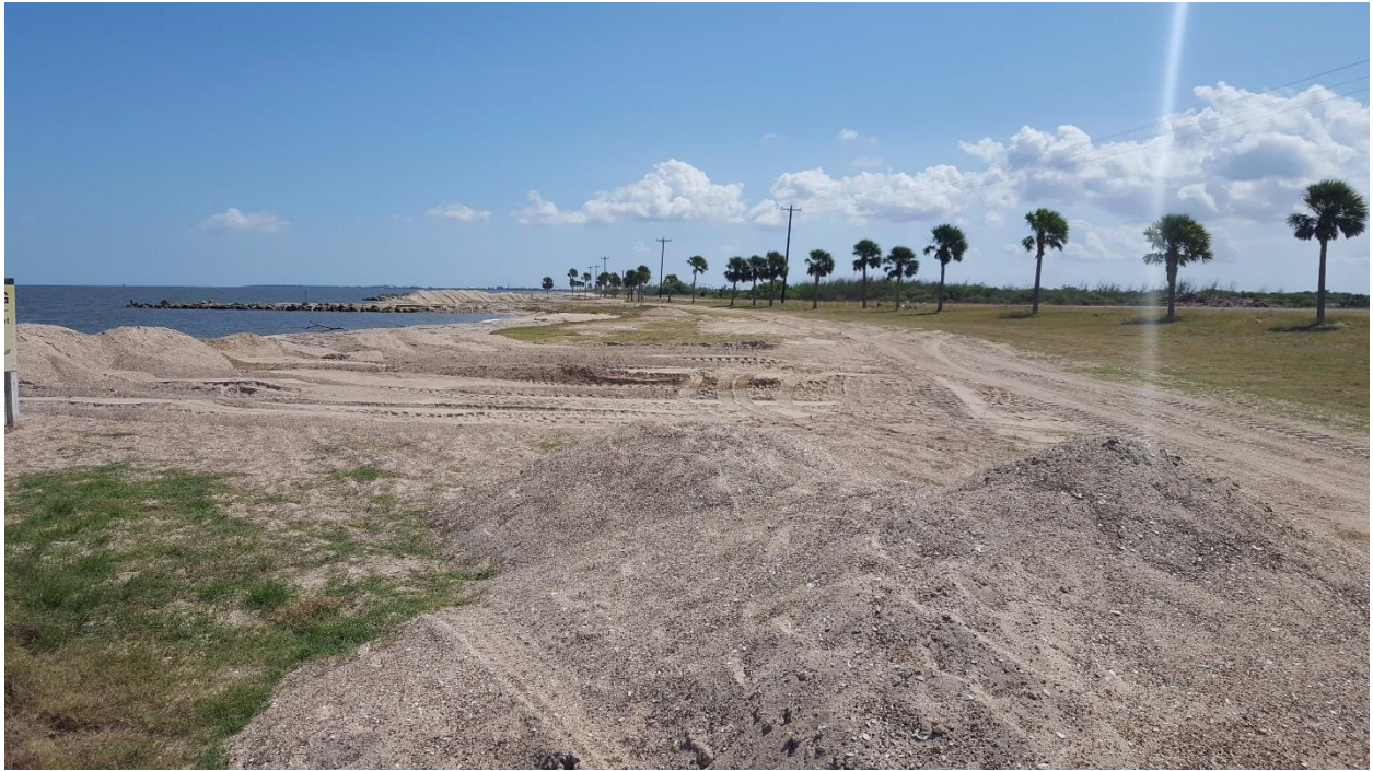
Southeast of STA 44+00
