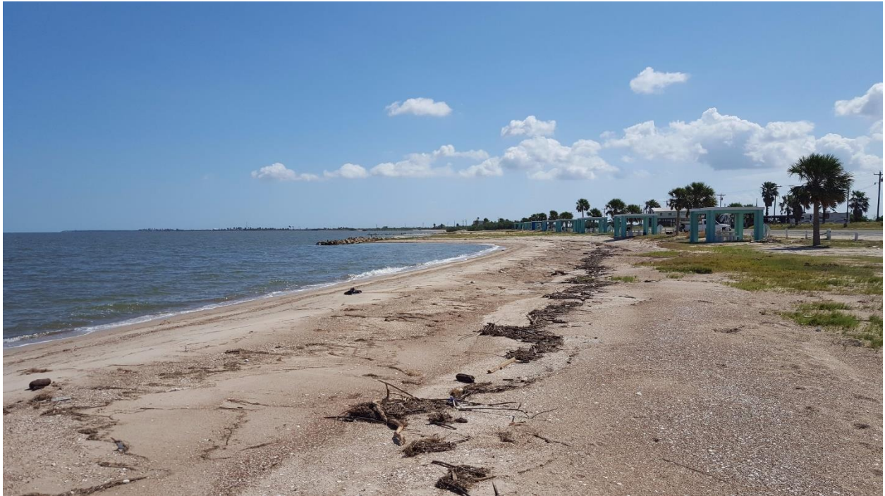
Southeast of STA 10+00
