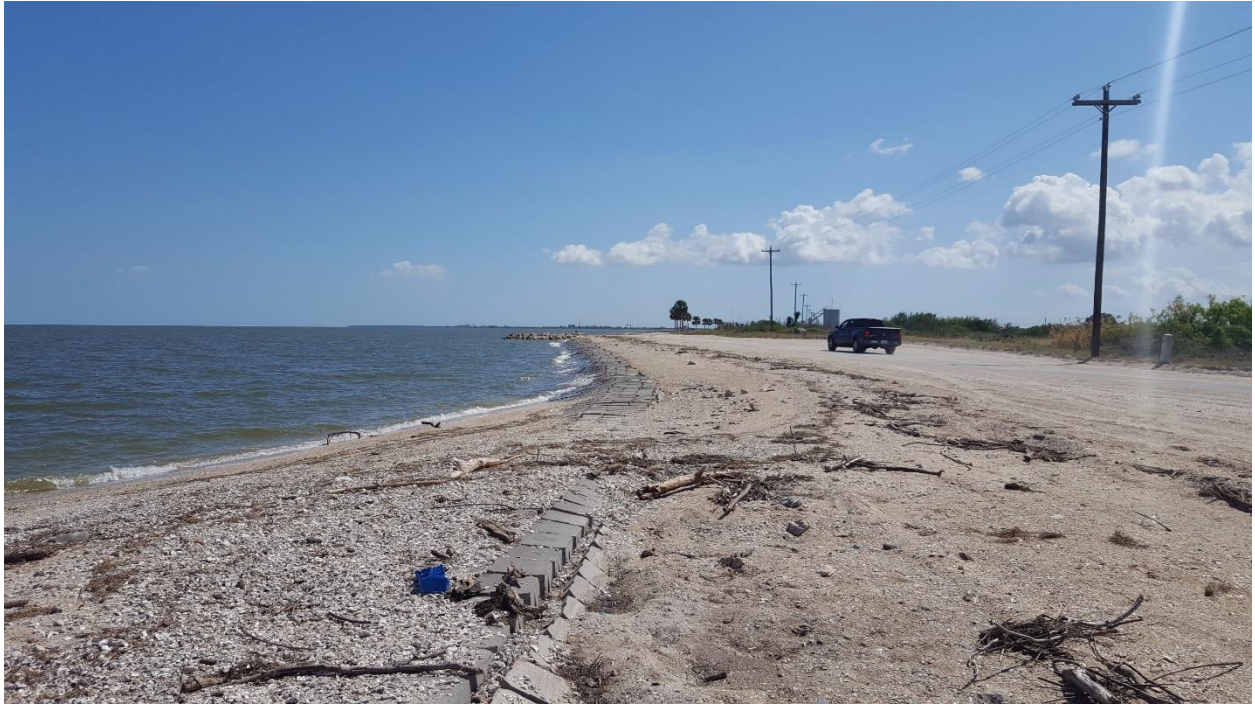
Southeast of STA 33+00
