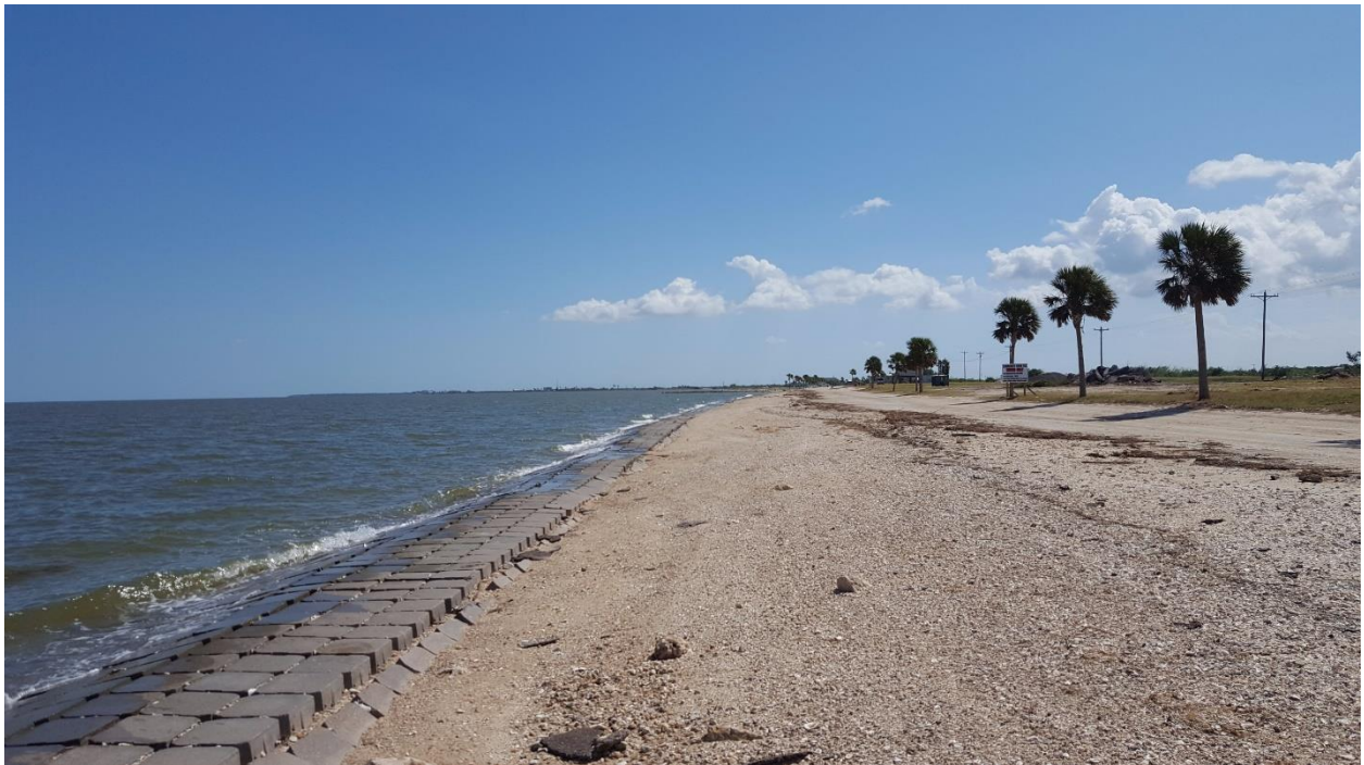
Southeast of STA 23+00
