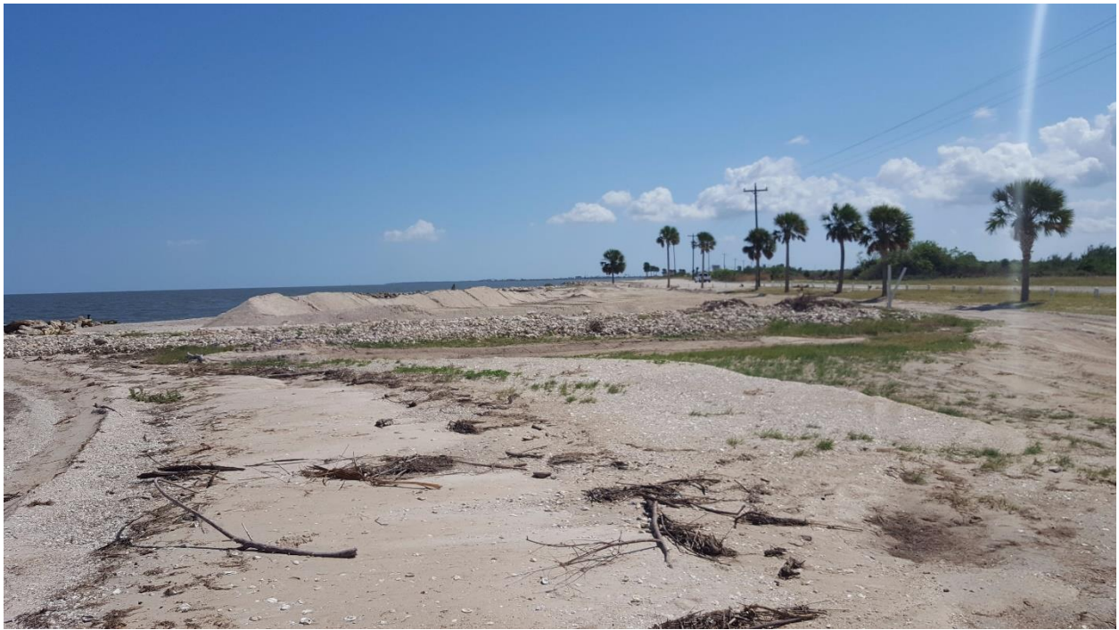
Southeast of STA 38+00
