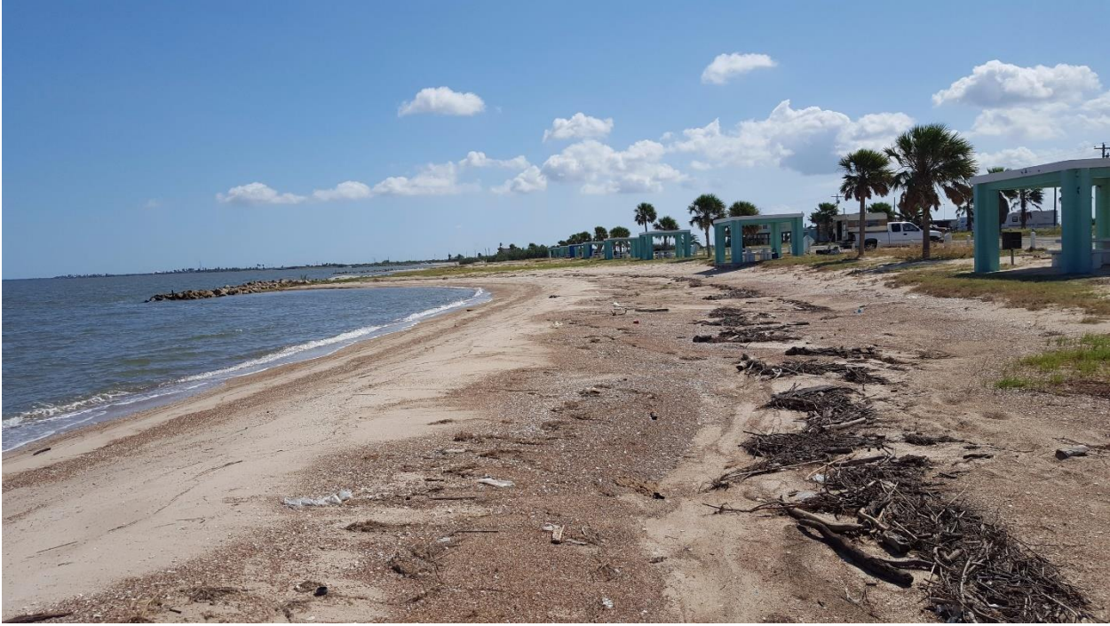
Southeast of STA 9+00
