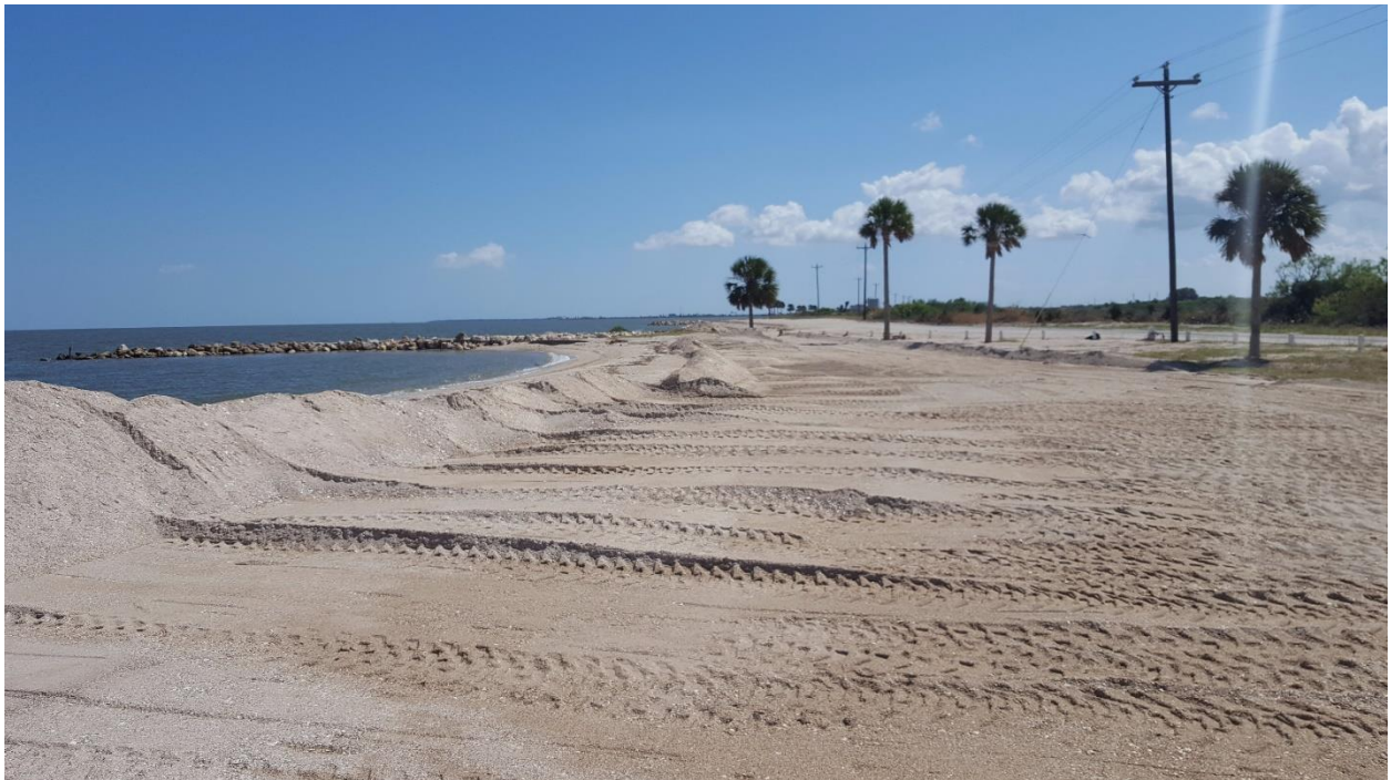
Southeast of STA 36+50
