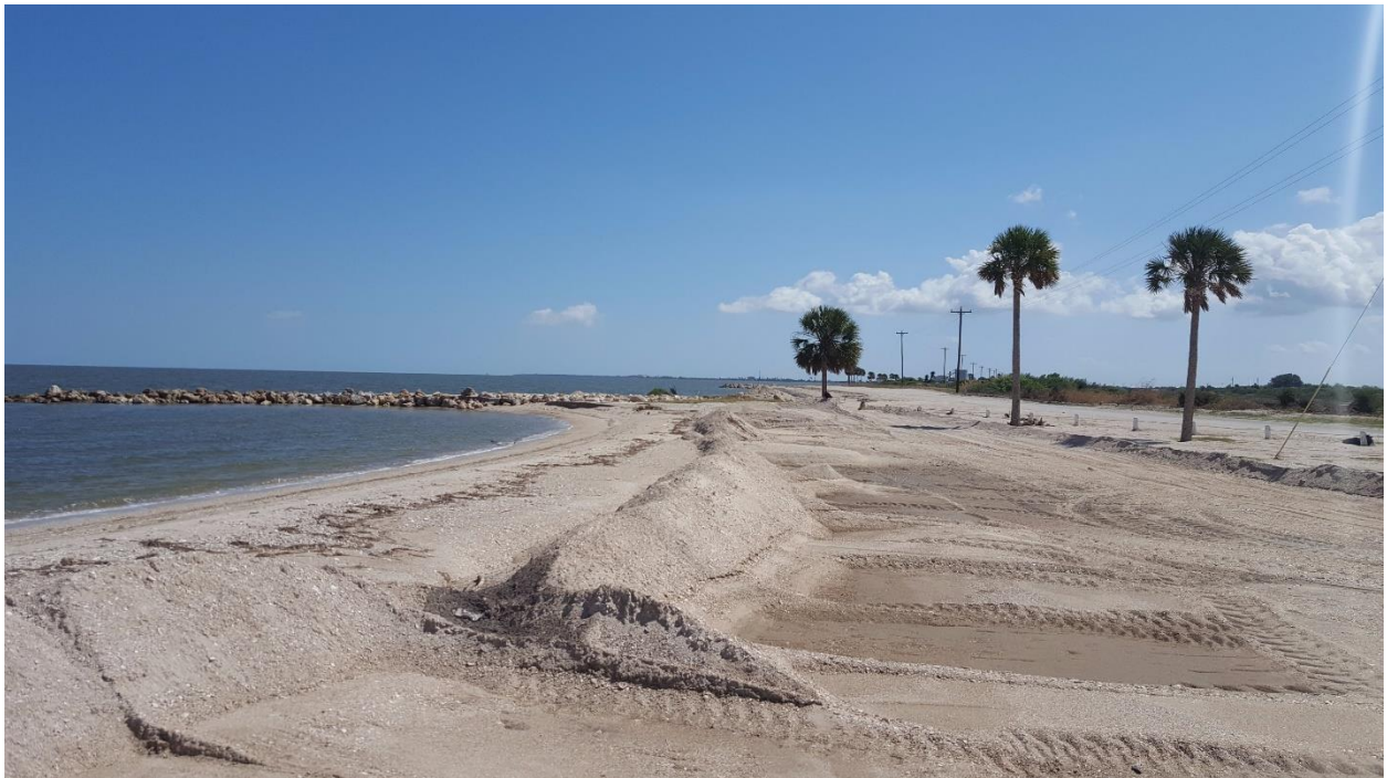
Southeast of STA 36+00
