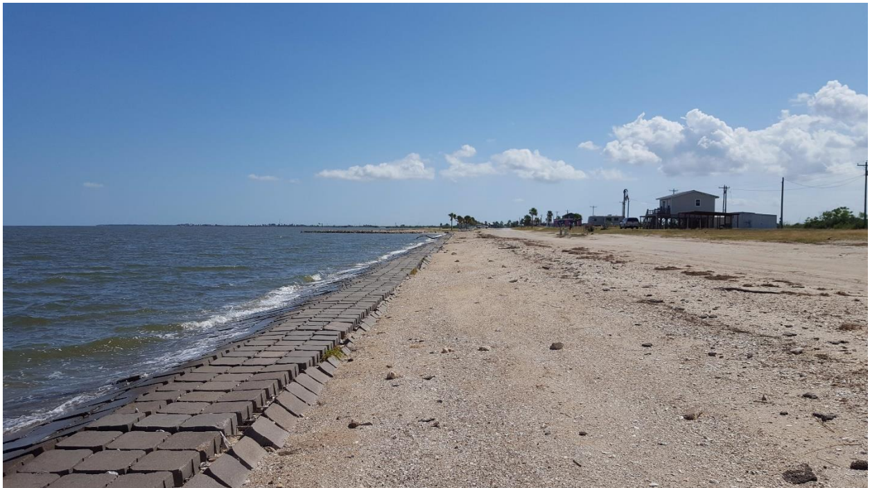
Southeast of STA 17+00
