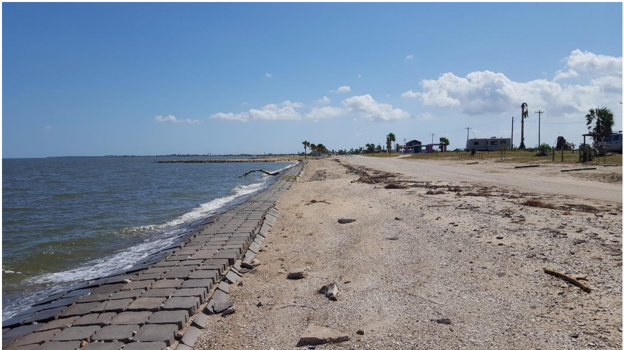
Southeast of STA 15+00
