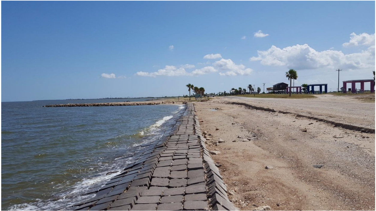
Southeast of STA 14+00
