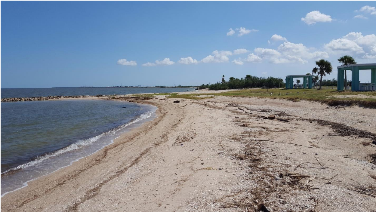
Southeast of STA 4+00
