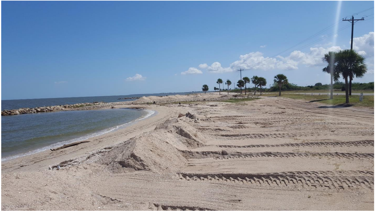
Southeast of STA 39+00
