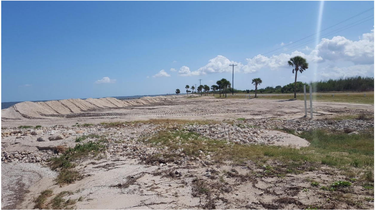
Southeast of STA 41+00
