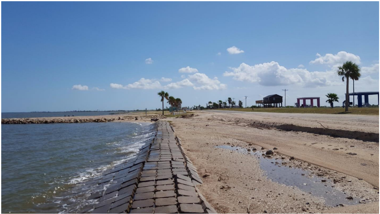
Southeast of STA 13+00
