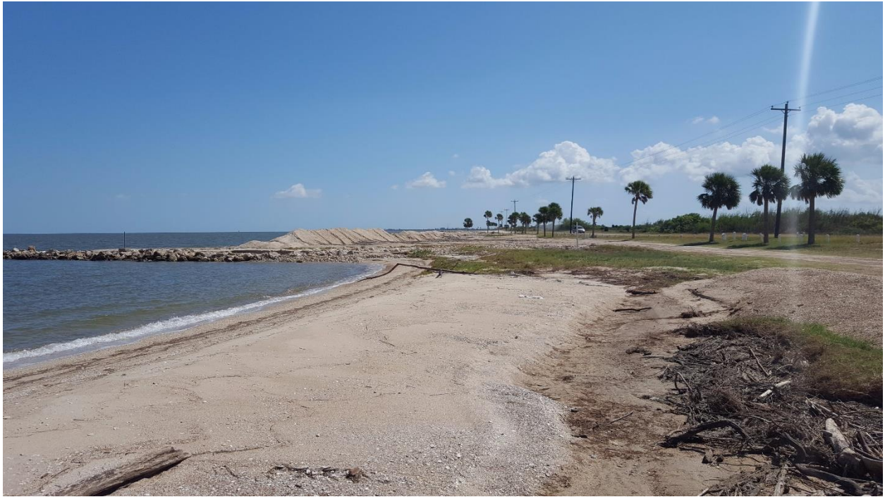
Southeast of STA 42+00
