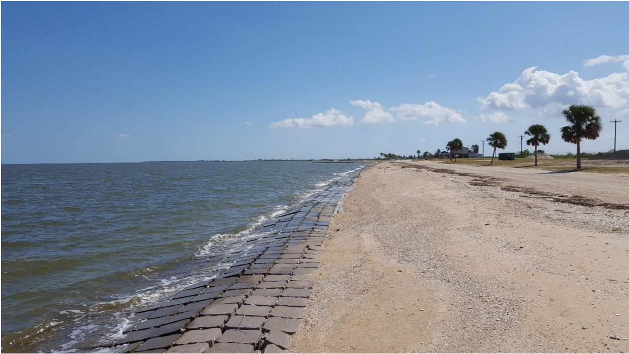
Southeast of STA 21+00
