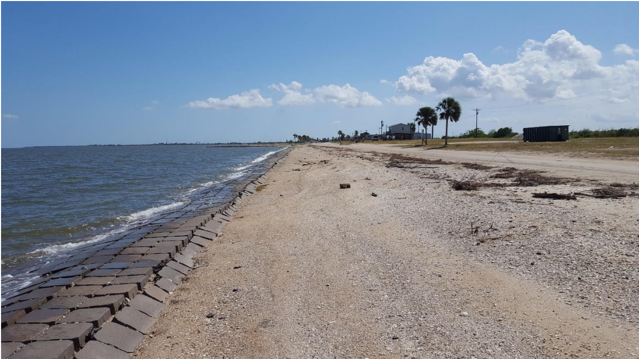
Southeast of STA 19+00
