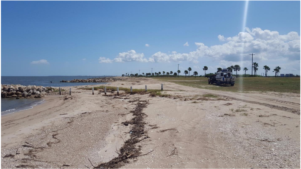
Southeast of STA 49+00
