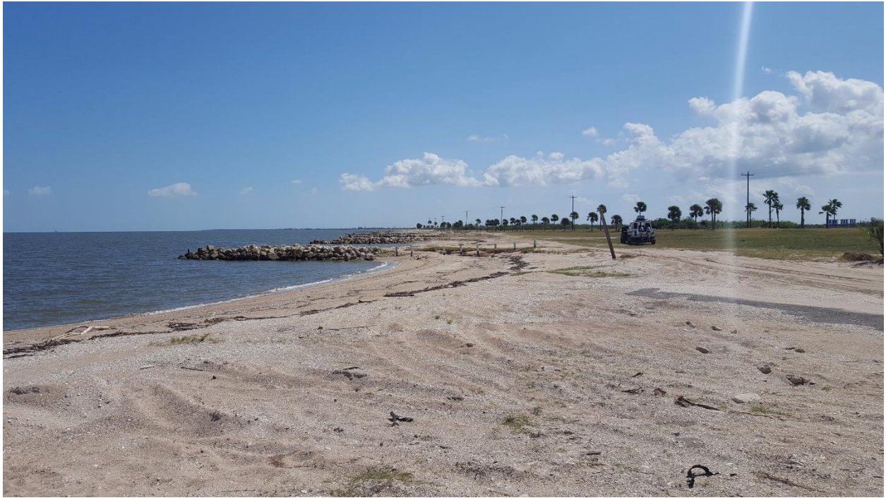
Southeast of STA 50+00
