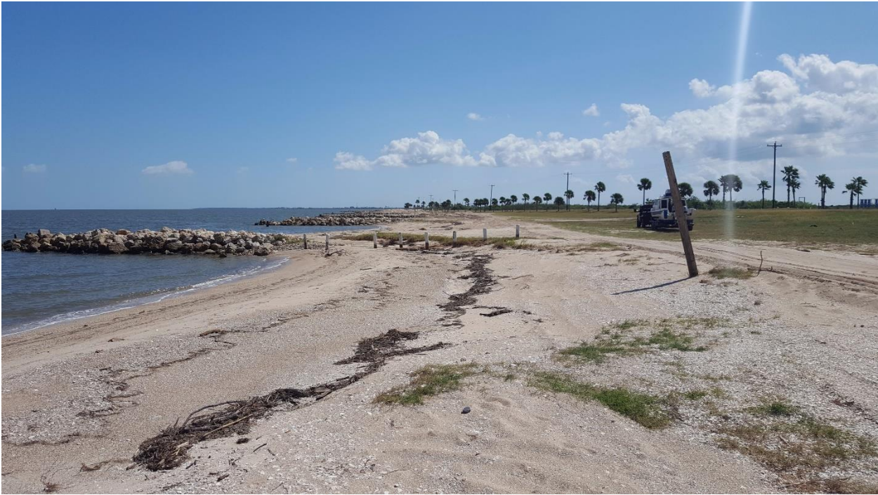
Southeast of STA 49+30
